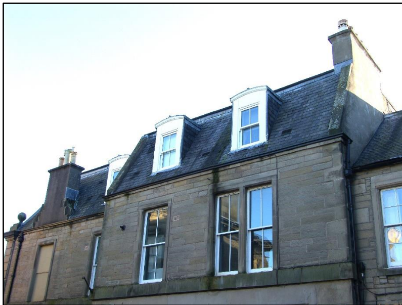
Steep-sided 'mansard' roof with dormer windows
