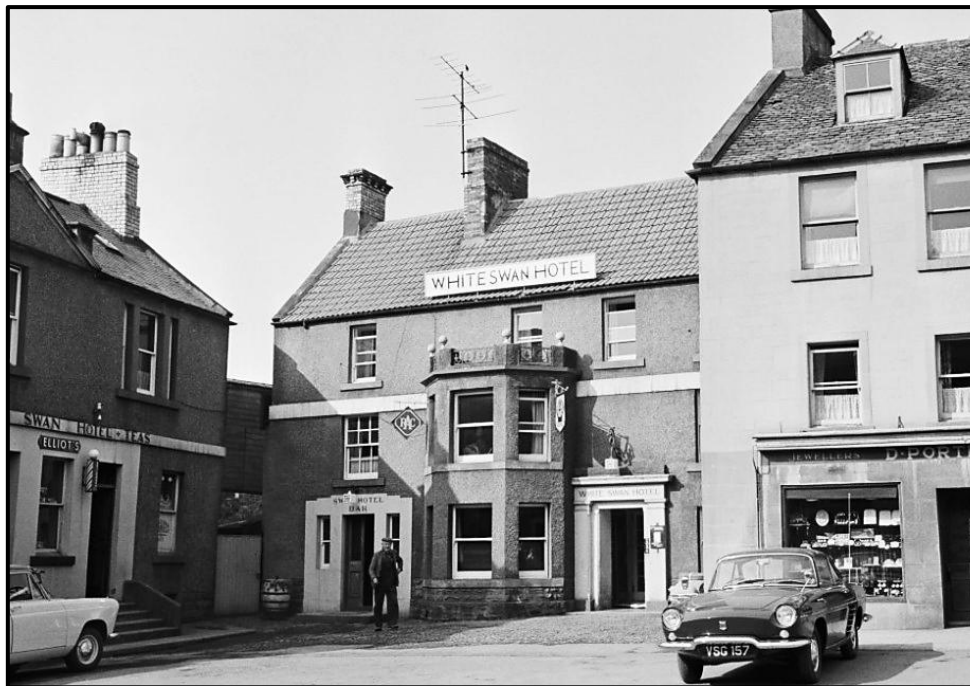
The White Swan Hotel in 1962 (© Crown Copyright : HES)
