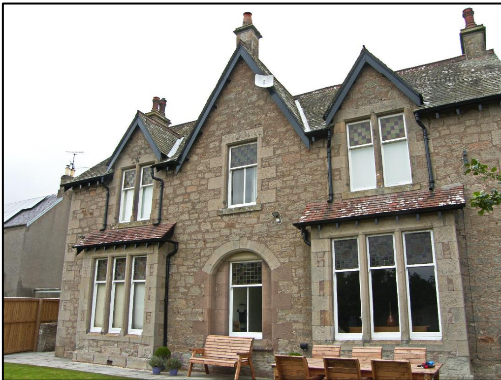
South elevation of Fenton Lodge : stained glass in all the upper panes
