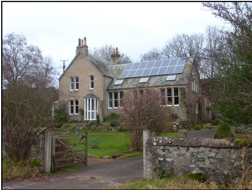
The 'new' Millburn schoolhouse (left) and schoolroom, opened in 1877
