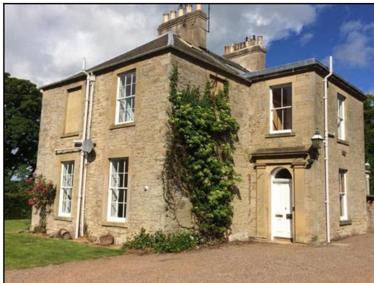
Rear entrance porch added by 1857
