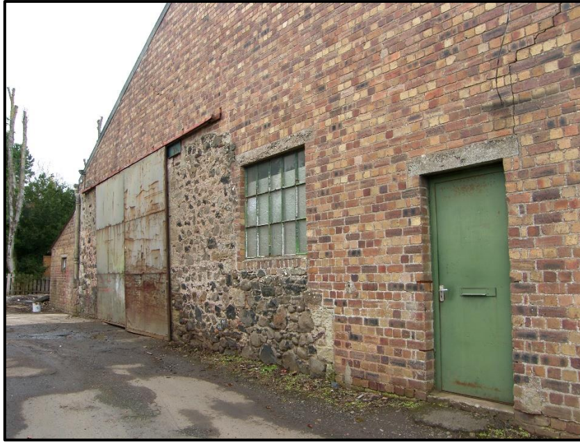
Evidence of the original stone and later brick construction
