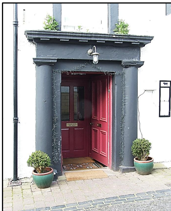
Plain Doric doorway with pilasters either side
