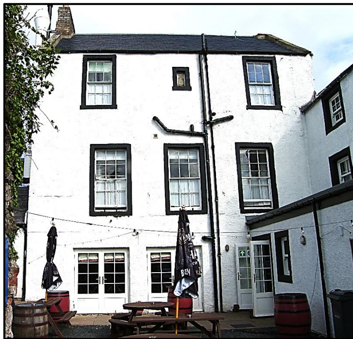
South courtyard elevation still retains the hotel's coaching inn character
