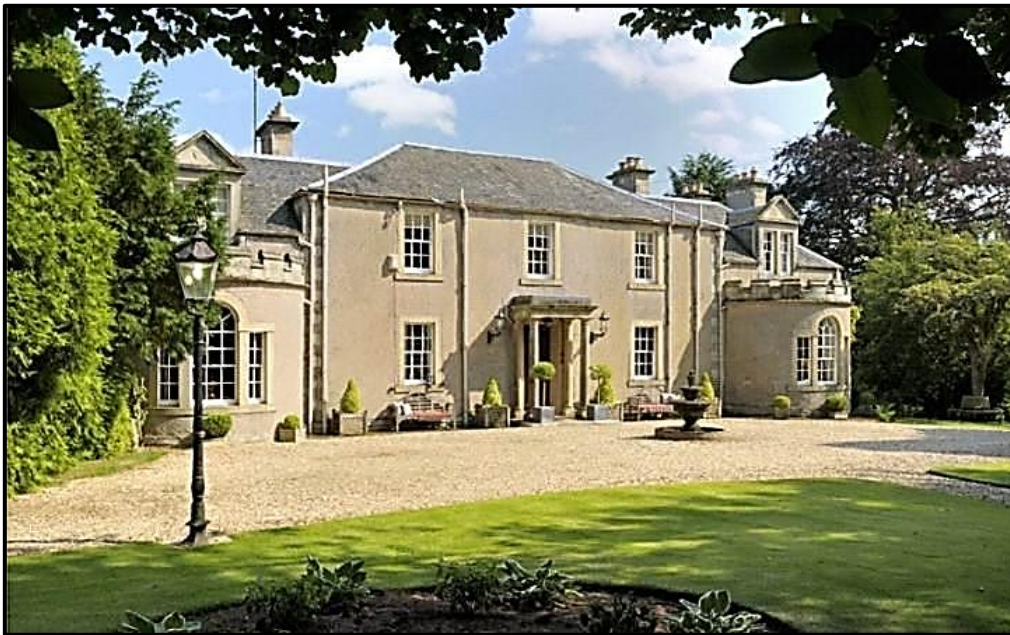
Wellfield's north (actually front) elevation
