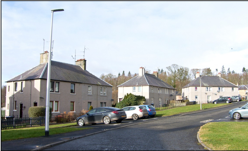
Part of the Earlsmeadow scheme, built by Duns Town Council in the 1930s
