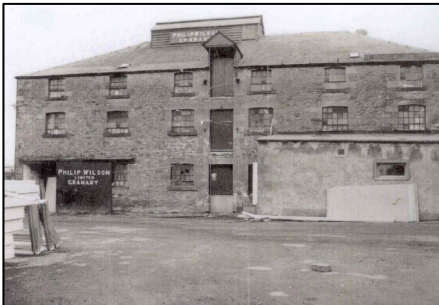
Wilson's station granary, destroyed by fire in 2021 and now demolished
