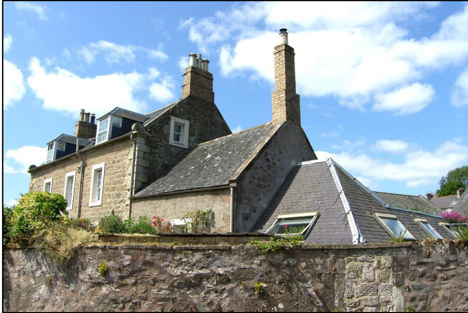
Evidence of various additions and alterations at Mansefield
