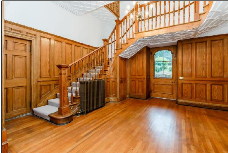
Timber panelling and ornate plaster ceilings at Wellnage
