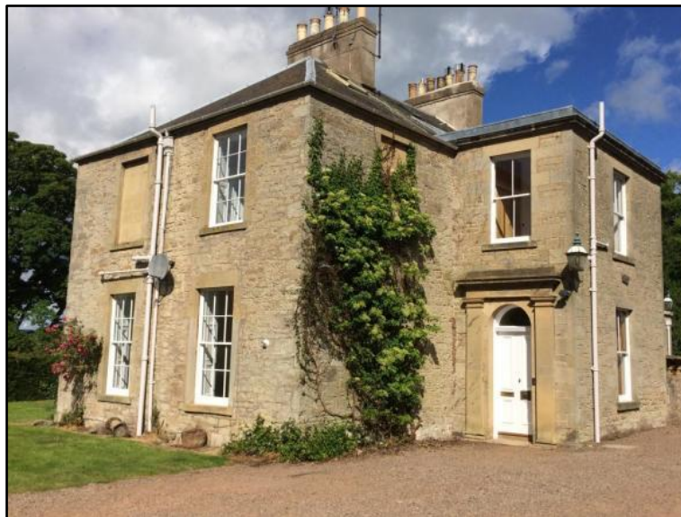
Rear entrance porch, added by 1857
