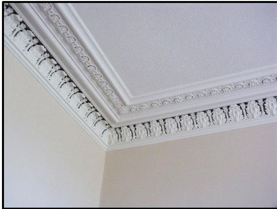
Original plaster cornice and timber fireplace detail at Kirkwell House
