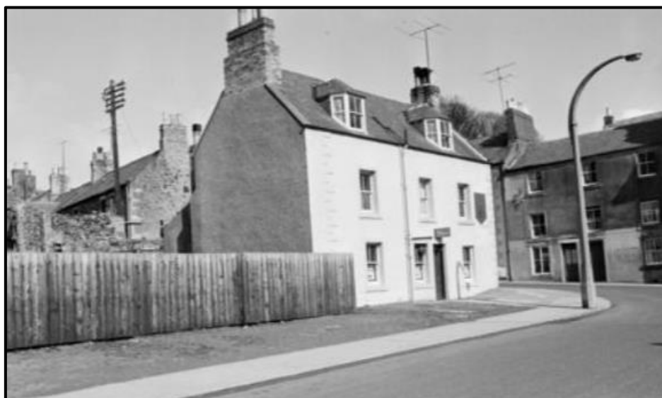
Gap site between County Buildings and Horn Inn caused by demolition of old domestic properties in 1938 (photo Canmore 1962)
