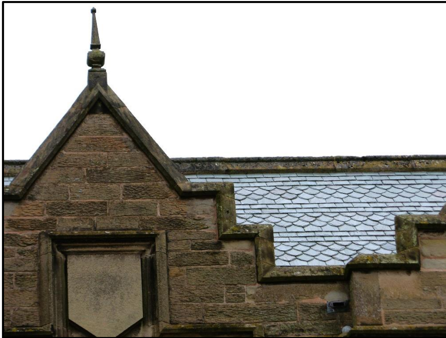
Dutch gable with finial and fish-scale slates at County Buildings
