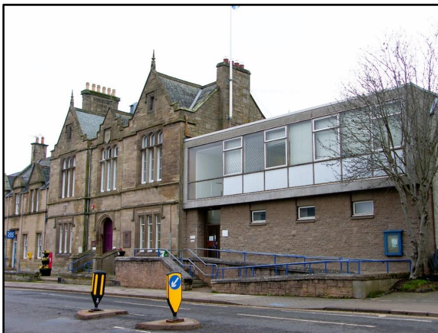
Flat-roofed extension built on gap site in later 1960s
